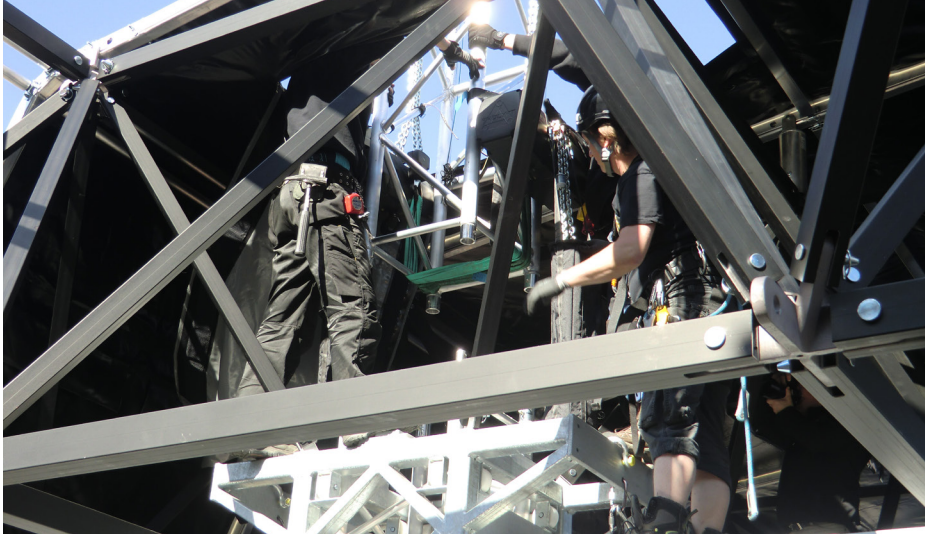
Photo: Space Roof Training Scenbyggarna
